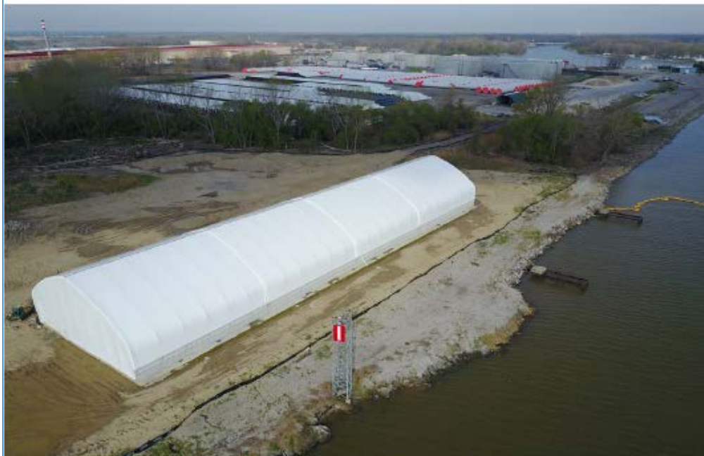
After Site Preparation and New Storage Building
