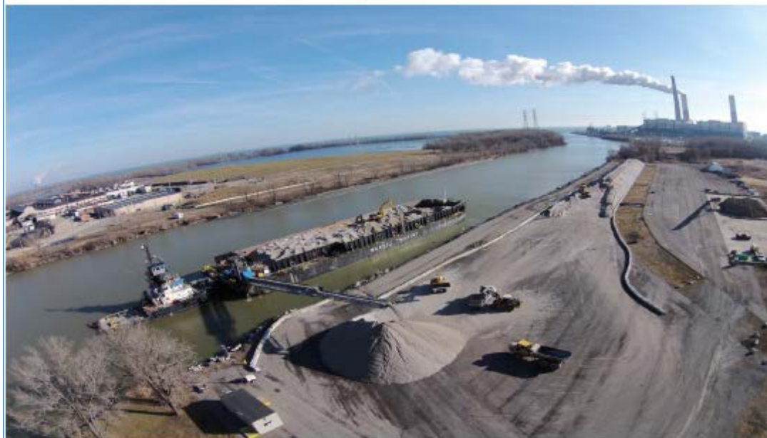
After Site Preparation - Dock Area
